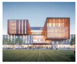
to be U of T Mississauga's first LEED Gold status structure—a recognition of achievement in energy and resource-efficient buildings. Design features will include: natural ventilation of the main public spaces to provide improved indoor air quality; elevated roof gardens and terraces overlooking the redesigned Campus Green area (formerly the north field) for faculty and student events; and solar shading.
